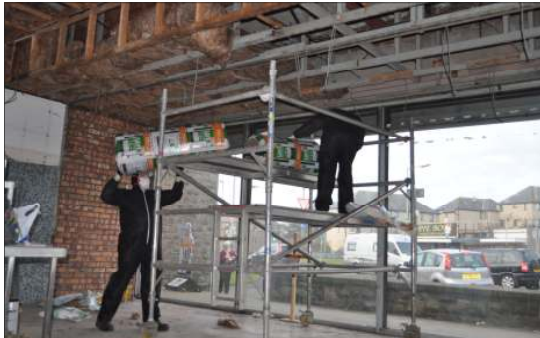
Insulation being installed in the roof space
