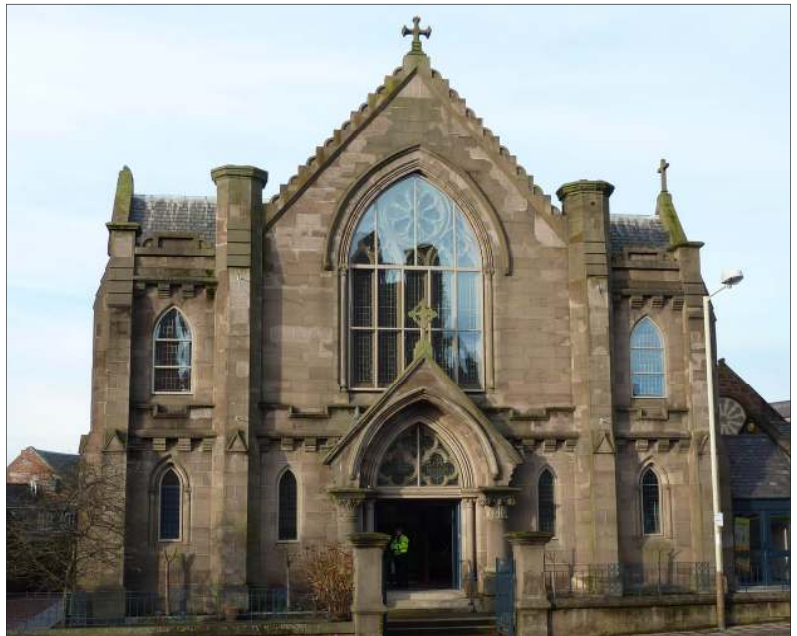
The Jean Glen Legacy Pictured above are the new double-glazed windows which have 'modernised' the frontage and received much positive comment.
