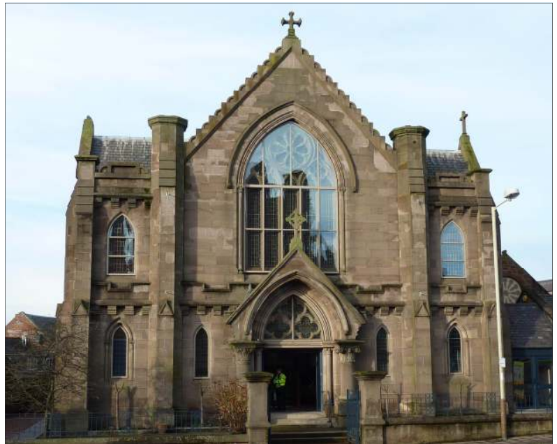
The Jean Glen Legacy Pictured above are the new double-glazed windows which have 'modernised' the frontage and received much positive comment.
